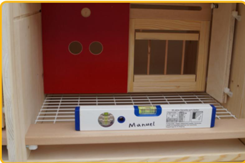
It must now be aligned using the spirit level and securely screwed to the back wall.
