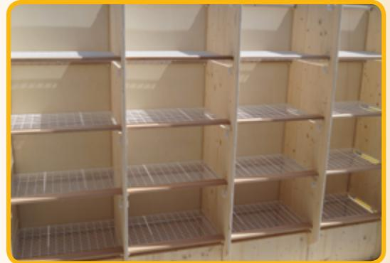
Now the wire meshes are inserted. The folds must point downwards.
