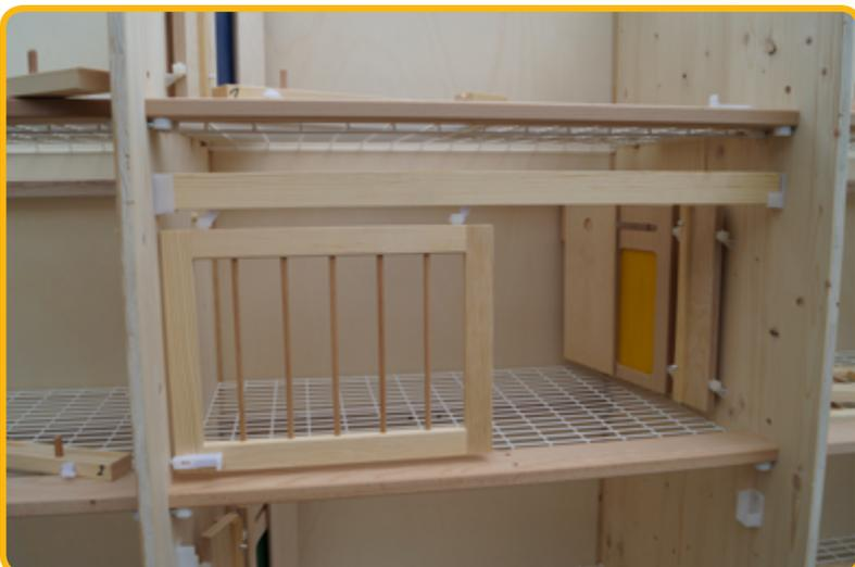
Fit the front bars with the front doors attached into all of the sections.
