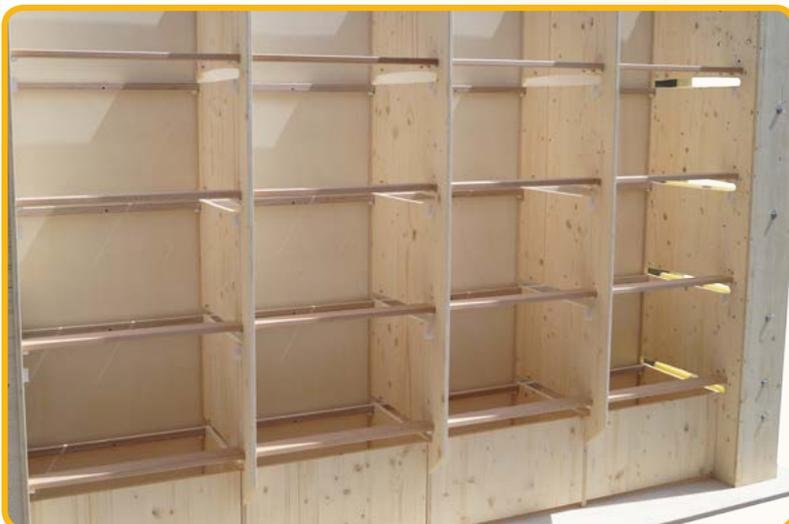
Press the beech wood perch bars onto the metal bolts on the upright side panels. 4 pieces per section. In doing so the notch on the bars must always point to the back.
